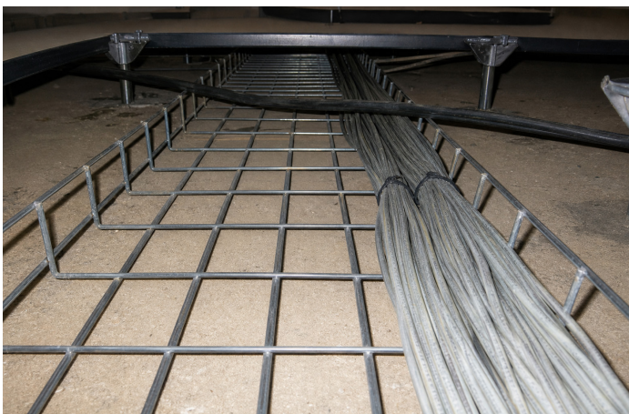
Data cable in tray with power cable running diagonally across the room.
