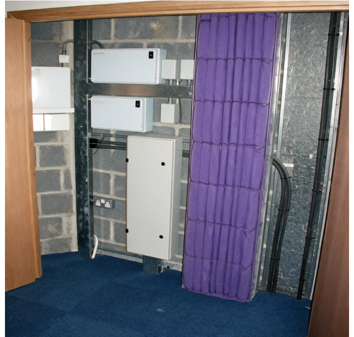
Data cable in tray with power cable running diagonally across the room.
